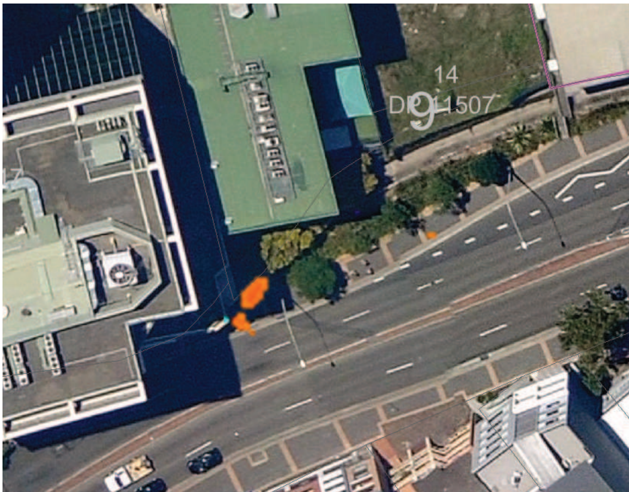
Figure 4.13: Parkes Street overland flow/open channel interface – Water Level Greater than 10mm
